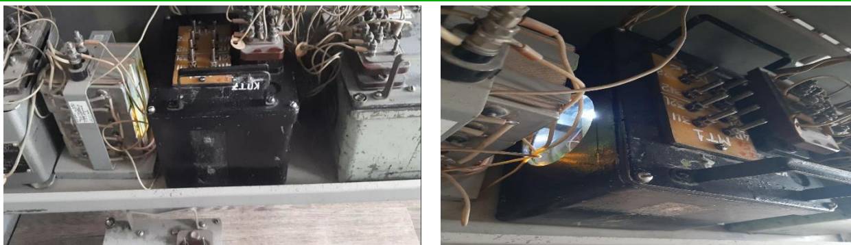
Figure. 2. Hamza station, connection of a microelectronic transmitter instead of КИТШ-5 and КИТШ-7
